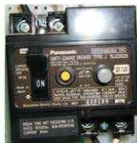
Figure: 2 Earth Leakage Circuit Breakers (ELCB) (Picture Courtesy Wikipedia)
