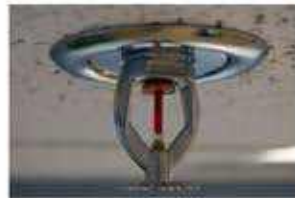
Figure: 22 Water Sprinkler (Picture Courtesy Google)
