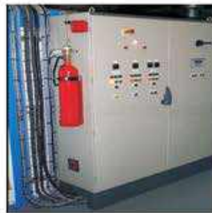
Figure: 4 CO 2 fire extinguishers, placed near major electrical panels (Picture Courtesy Wikipedia)
